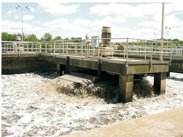
Figure 8.6 Secondary treatment
